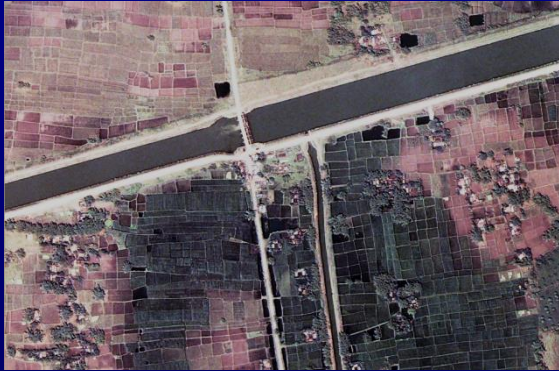
Completed section i.e., canal in place
