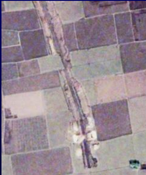
Canal under construction
